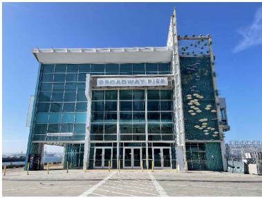
EXTERIOR FACADE (LOOKING WEST)
