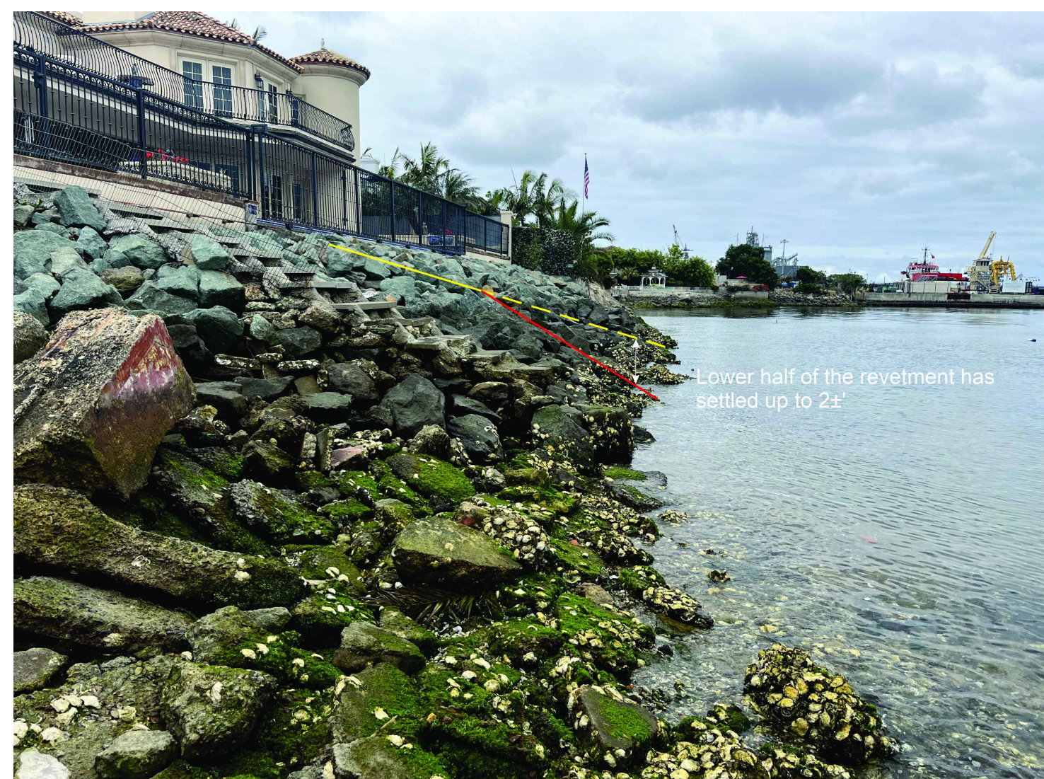
PHOTO 1, LOOKING NORTHWEST AT EXISTING REVETMENT FRONTING 407 1ST STREET. NOTE LOWER HALF OF THE EXISTING REVETMENT HAS SETTLED CAUSING A STEEPENING OF REVETMENT FACE.
